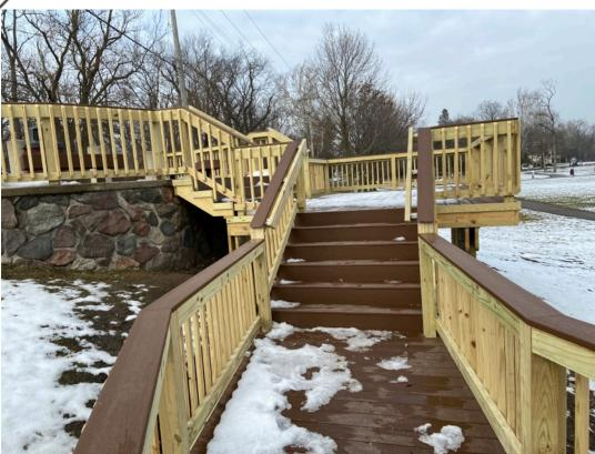
The stairway leading down to Congdon Park has been replaced, using mostly composite wood that will not need to be stained. It will be power washed in spring. A few additional additions like an area to the bottom left of the staircase will be added to provide an area for future additions to existing memorable plants, benches, etc.
